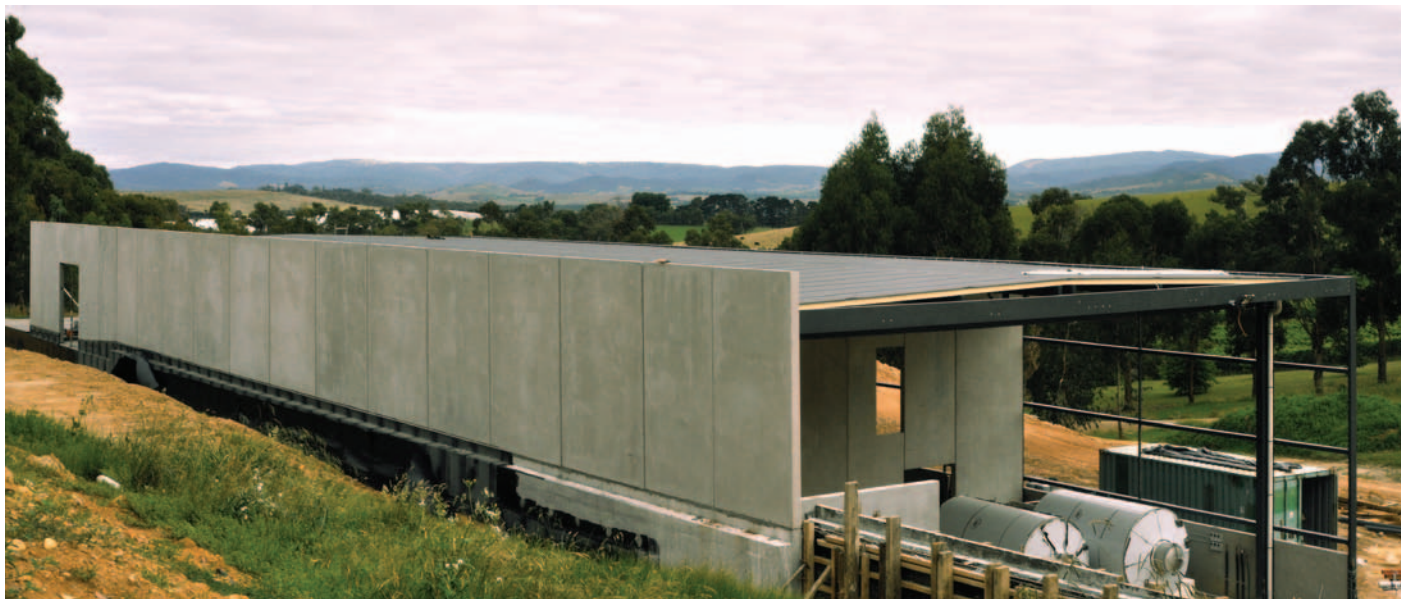
Medhurst Winery, photographed from the south-east angle, showing the main wall and what will be the vintage area. It was 6 weeks from completion and first vintage.
