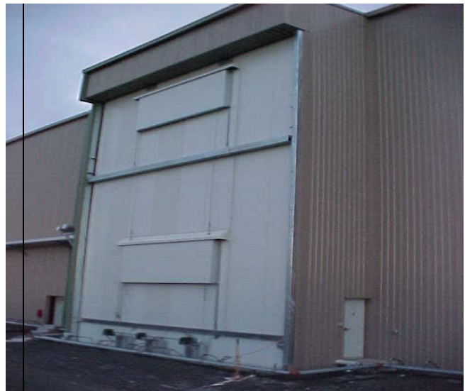
Figure 12 – External view of alcove showing defrost doors in the closed position, with personal access door at side.
