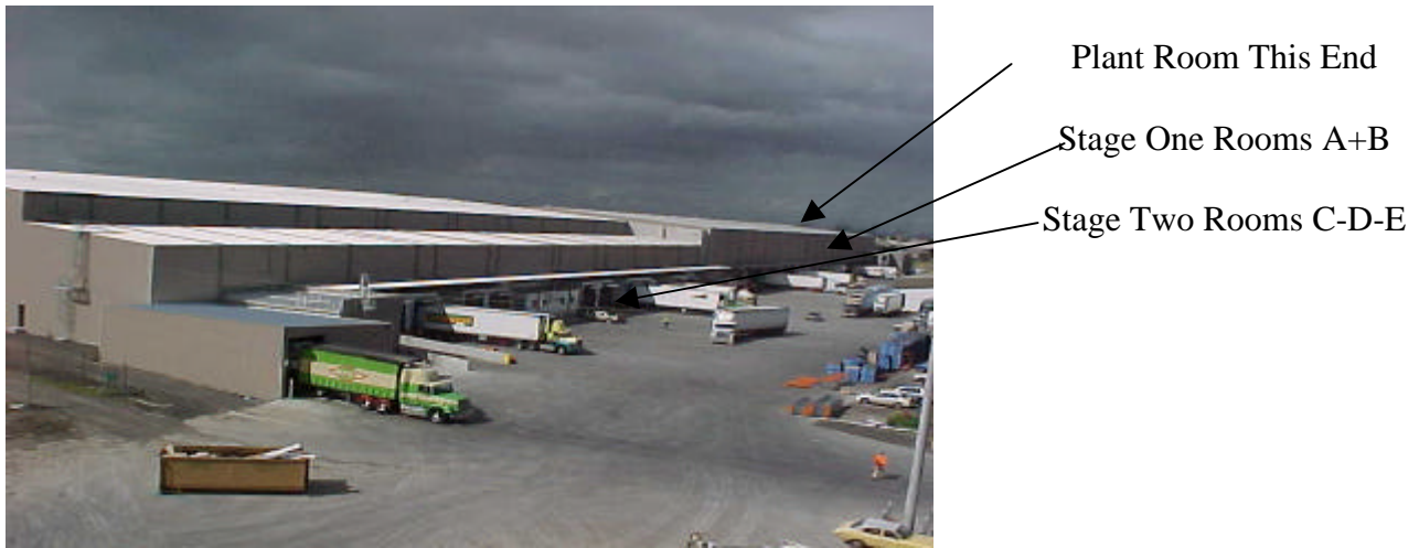
Figure 1 – Cold Store Extension, Melbourne Australia.
