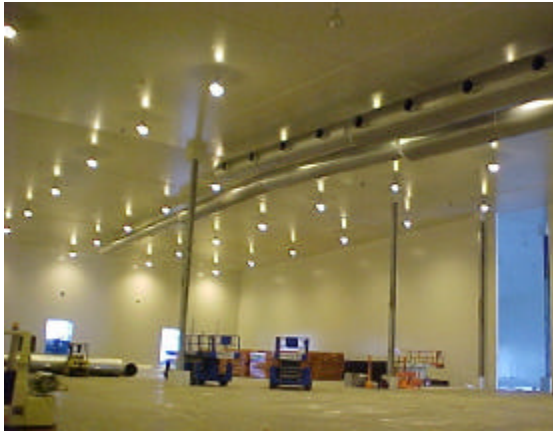
Figure 2 – Freezer room during installation showing air distribution ducts.
