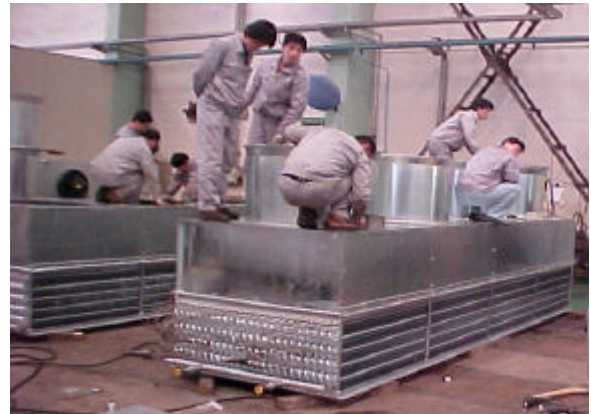
Figure 9 – Ammonia air-cooling evaporator under construction.
