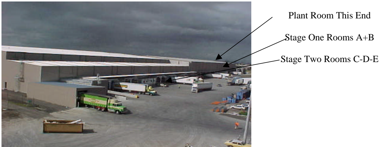
Figure 1 – Cold Store Extension, Melbourne Australia.
